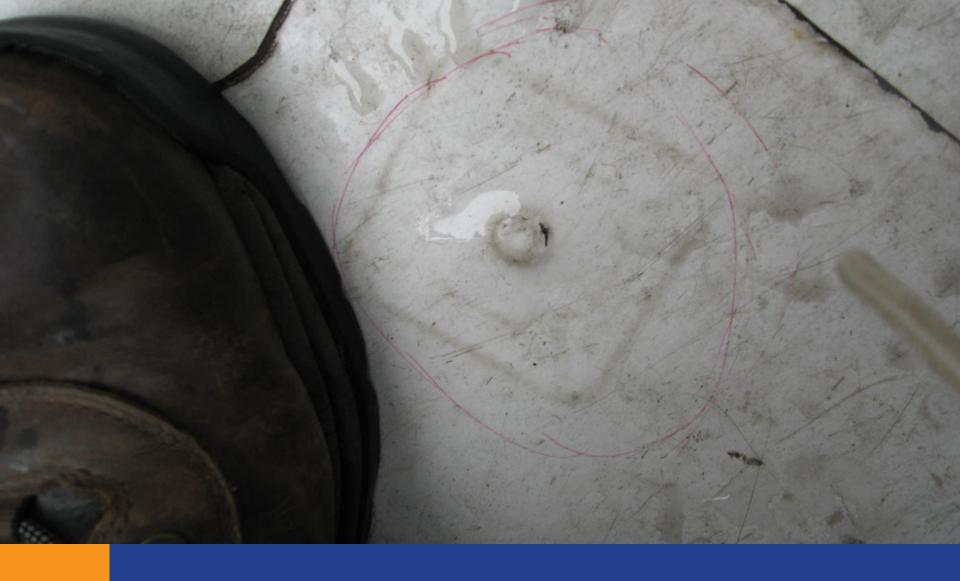
Fasteners Directly Under Membrane Cause Problems
