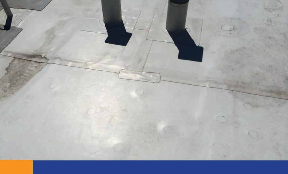
**Fasteners Directly Under Membrane Cause Problems**
